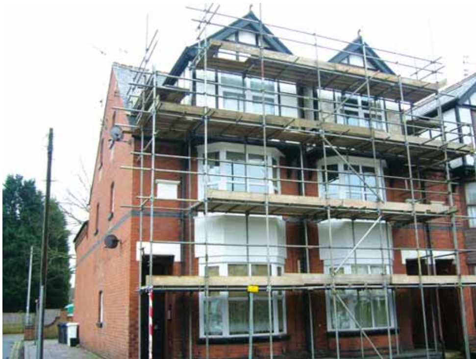
scaffolding erected for installation of UPVC double glazing
